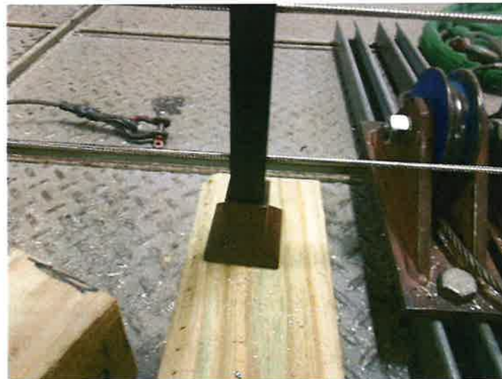
Photo No. 12 Support Baluster to Floor
