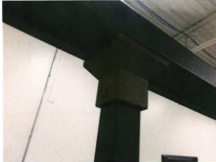
Photo No. 11 Support Baluster insert into Top Rail
