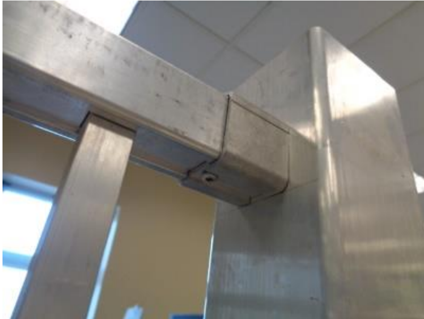
Photo No. 7 Top Rail Collar Bracket and Connections
