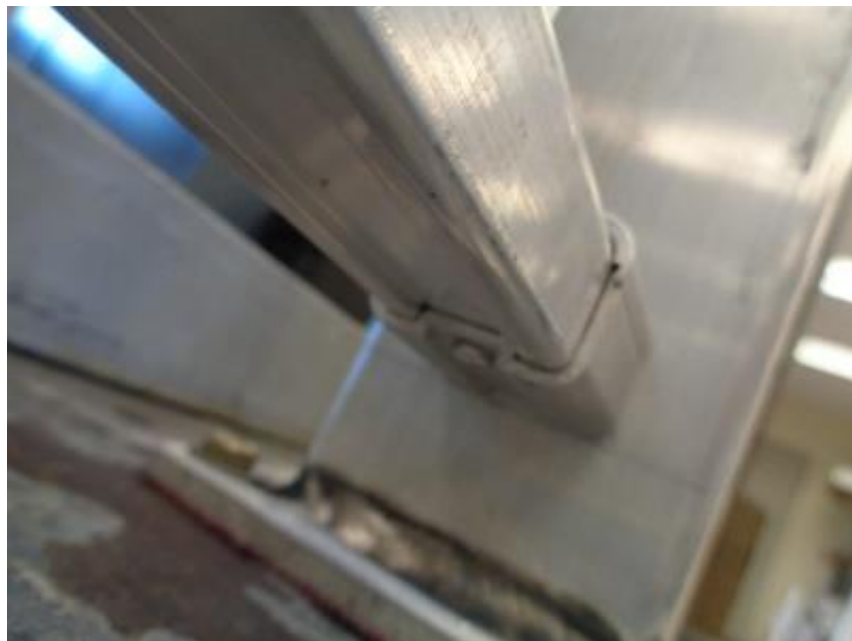
Photo No. 6 Bottom Rail Bracket and Post Mount Connection
